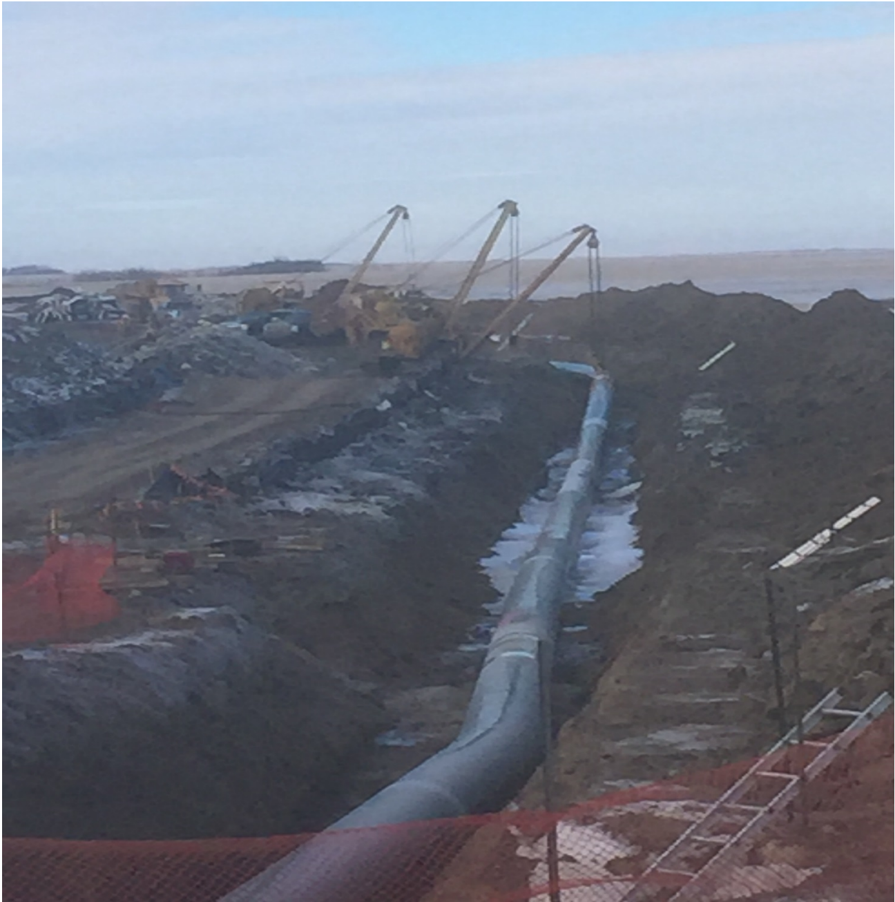
PIPE LAYING IN A TRENCH.
