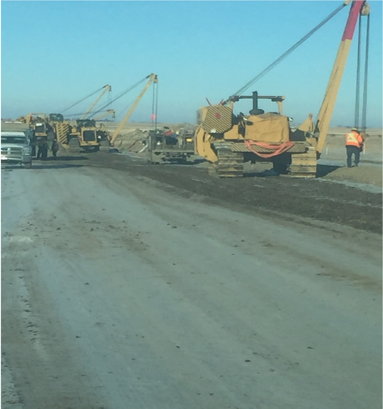
LOWERING PIPE INTO TRENCHES.
