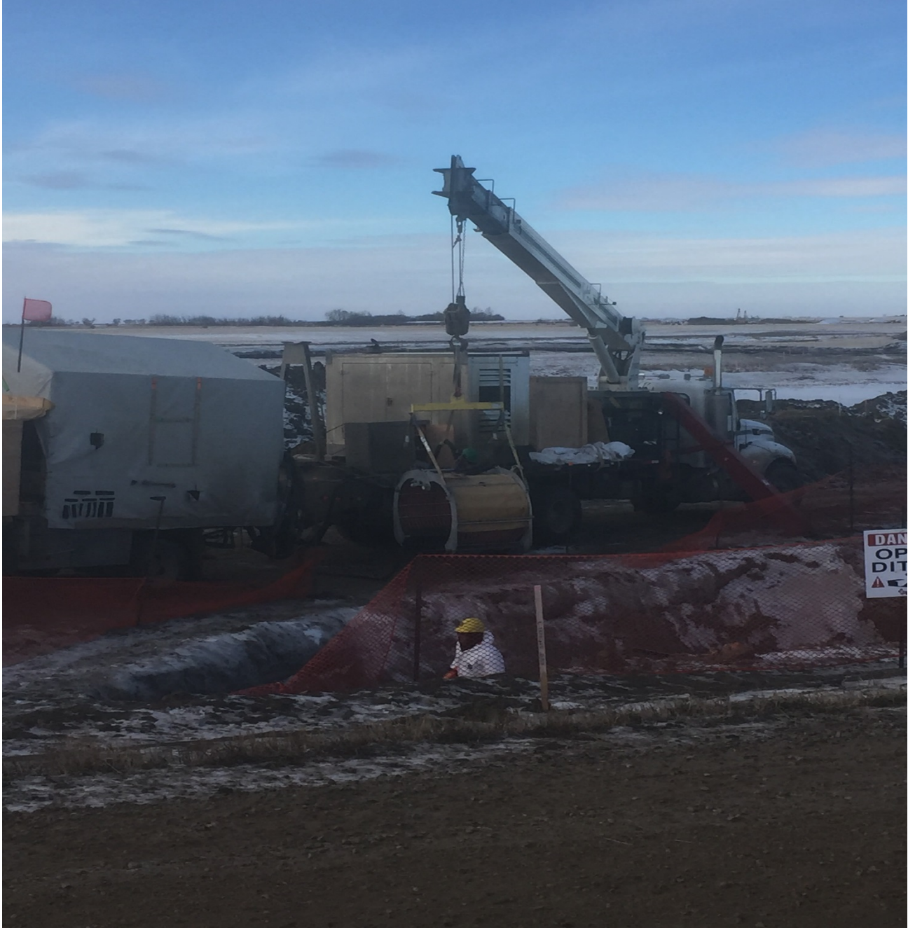
SANDBLASTING PIPE TO GET READY FOR COATERS.
